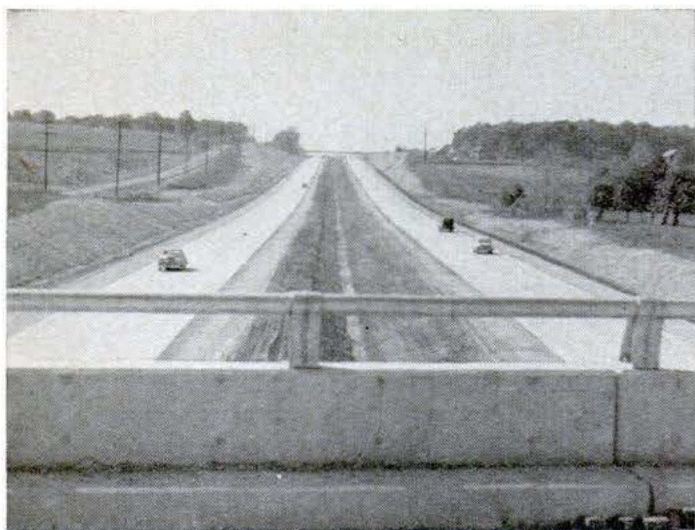
CENTER STRIP 56 feet and wider separates opposing traffic lanes of the Ohio Turnpike. A deep ditch runs down the middle portion.
